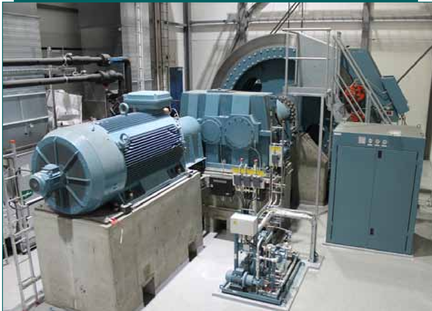
Figure 1 The multi-rope friction hoist at the Renström mine
